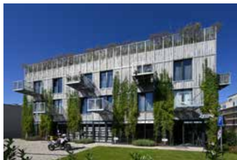
La Vida Residence, Praha / under- construction architects (2022)
